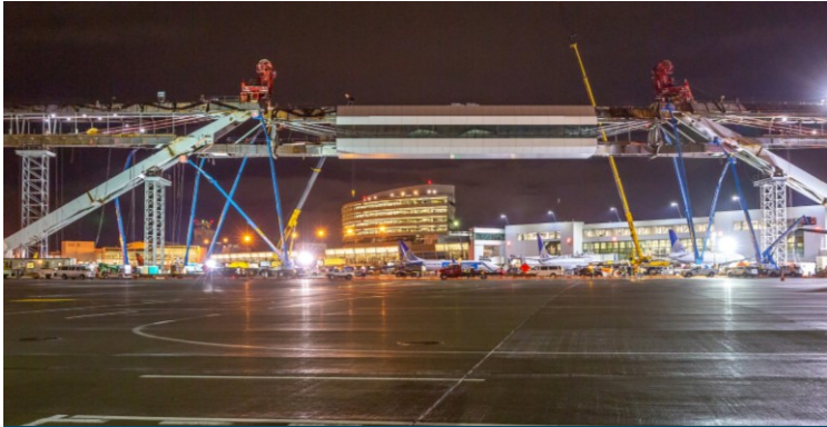
INTERNATIONAL ARRIVALS FACILITY
